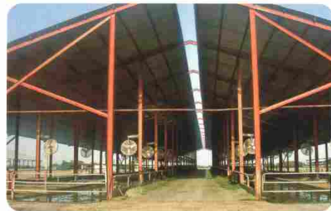
New barns are built. Sand is used as bedding
